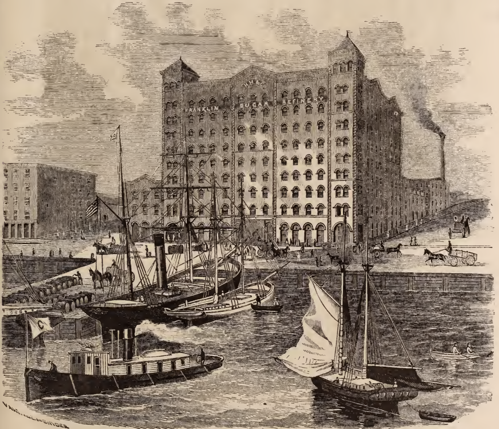
FRANKLIN SUGAR REFINERY.
